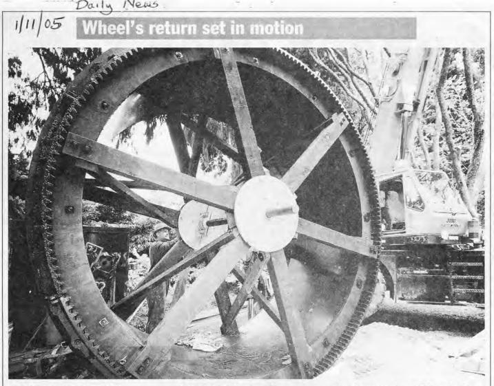
BIG WHEEL: Engineer Ken Kowalchuk cleans the shaft of Pukekura Park's new giant waterwheel in preparation for the fitting of bearings.
